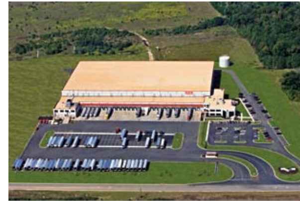
Personal vehicles and pedestrians (entrance at far right) never cross paths with truck traffic (entrance/exit second and third driveways from right) at the Sara Lee facility in Macon, Georgia, recently designed & built by Tippmann Group.
