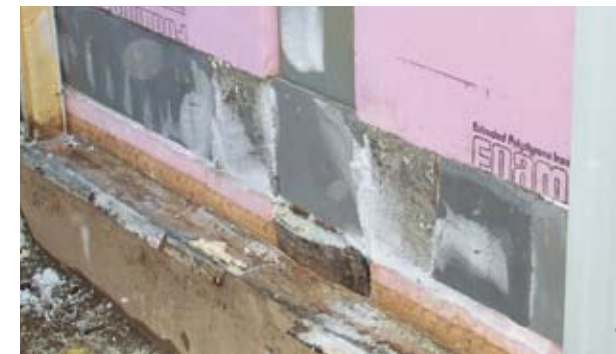
When oak blocks absorb moisture and freeze, they can swell and cause major damage to a warehouse.
